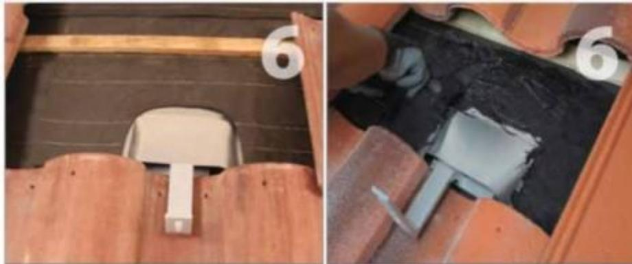
*To be code compliant, tile hooks must have metal flashing installed using Tile Roofing Institute approved underlayment bibbing (shown on the left). Three coursing with roofing cement and reinforcing fabric (shown on right).*
