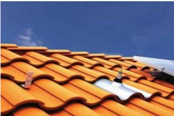
Roofs over 2:12 pitch are considered steep slope and instead of using a waterproofing membrane like a low slope roof, they typically use water shedding roof coverings that rely on gravity to keep the water out of the structure. The significant majority of steep slope roofs use asphalt shingles or tile. The other common steep slope roof options include
