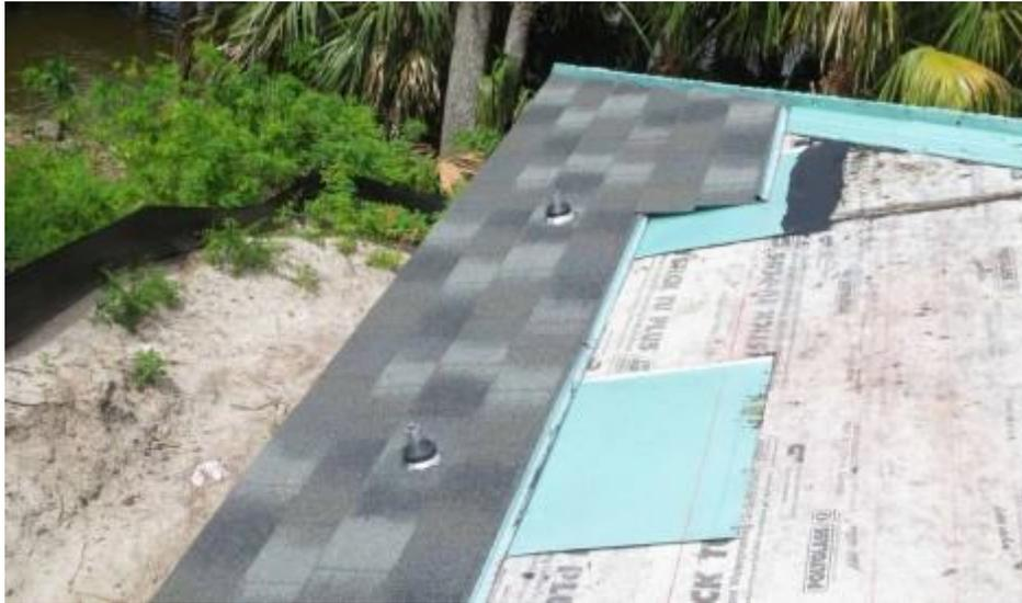
*This home with [Decra](#) metal shingles in Florida uses standoffs with flashing installed with a Decra “Underpan” to channel any leakage safely to the top of the shingles below.*
